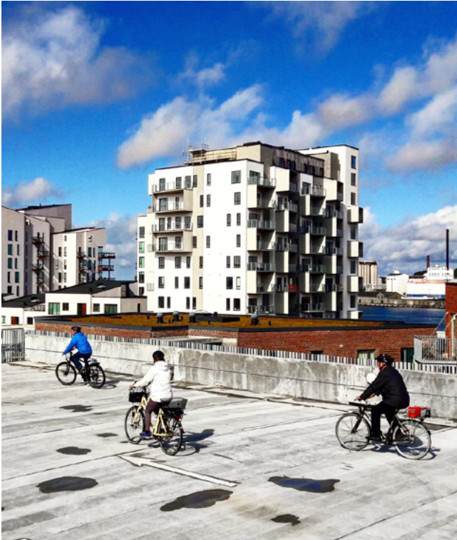
Bikes on the top of a newly constructed parking house at the Limfjord. Photo: Mike White.
