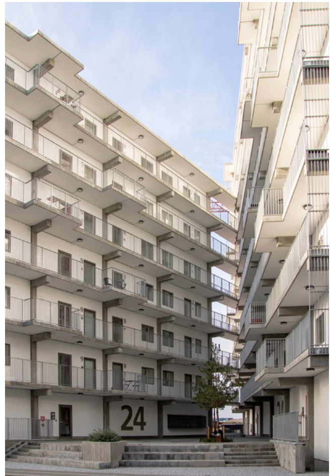
Building density in a new area of Aalborg. Photo: Inge Marie Møller Nielsen.
