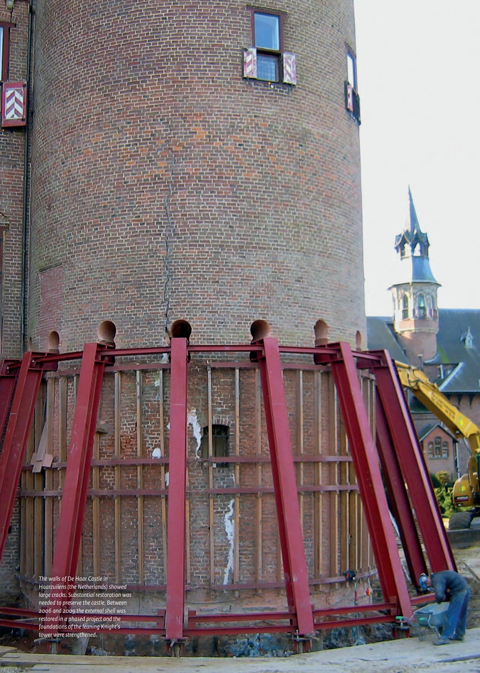
The walls of De Haar Castle in Haarzuilens (the Netherlands) showed large cracks. Substantial restoration was needed to preserve the castle. Between 2006 and 2009 the external shell was restored in a phased project and the foundations of the leaning Knight's tower were strengthened.
