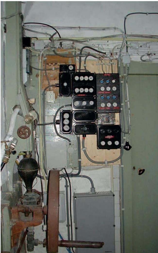
Figure 57. Fuse boxes: an electrical source of fires
