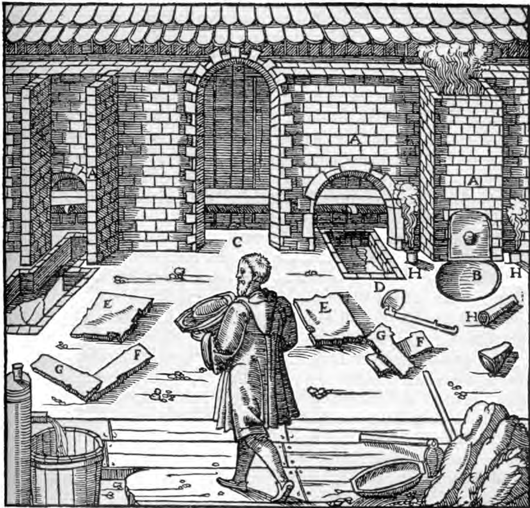
Smelteovner for kobbermalm. Tressnitt i Georgius Agricola: De re metallica (1556)
