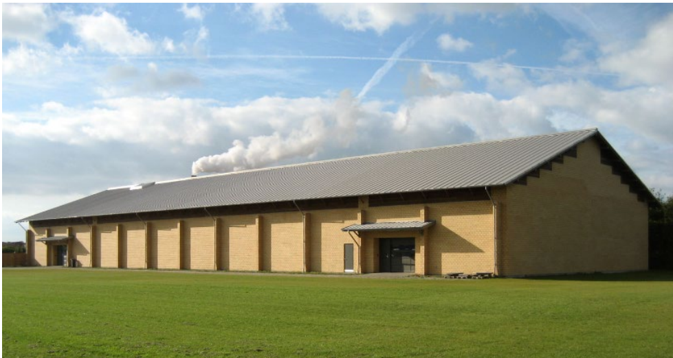
Figure 10. A purpose build storage for a collection of cultural history, Ribe, DK. The concrete floor has no thermal insulation to allow thermal buffering by the ground. The thermal insulation in the ceiling and walls is designed to allow an annual temperature variation between 8 °C and 16 °C. Photo: Poul Klens Larsen.
