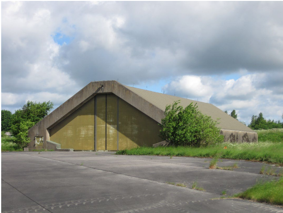
Figure 8. A solid concrete shelter reused for temporary storage of furniture. The roof thickness is 0.5 m and it has no thermal insulation. Værløse Airfield, DK. Photo: Poul Klenz Larsen.
