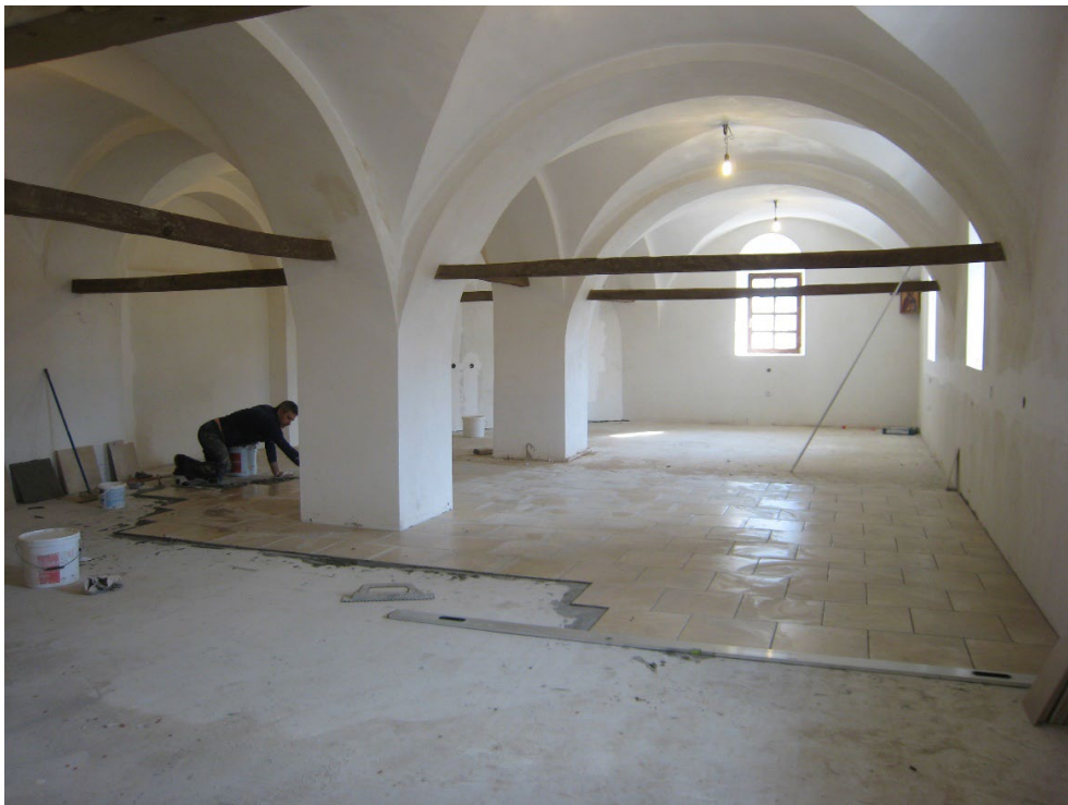
Figure 23. Heavy walls and ceilings have a large thermal inertia, which can even out the daily temperature fluctuations, but not the change in temperature from winter to summer. New library, Zografu Monastery, Mount Athos, Greece. Photo: Poul Klens Larsen.
